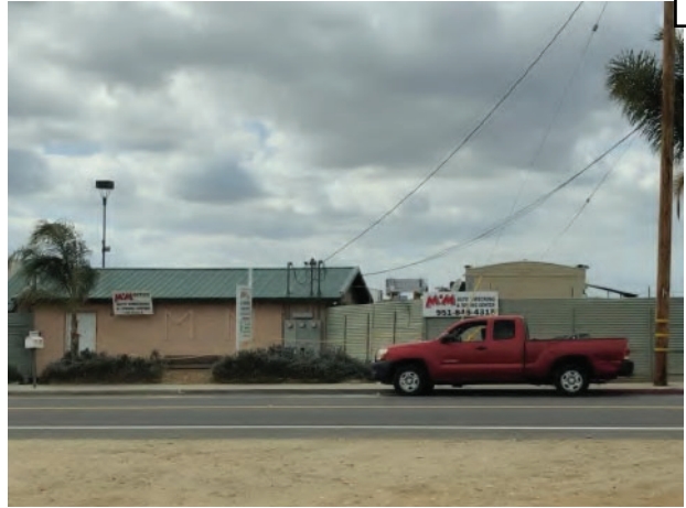
26.View of the adjacent auto-wrecking yard to the west.
