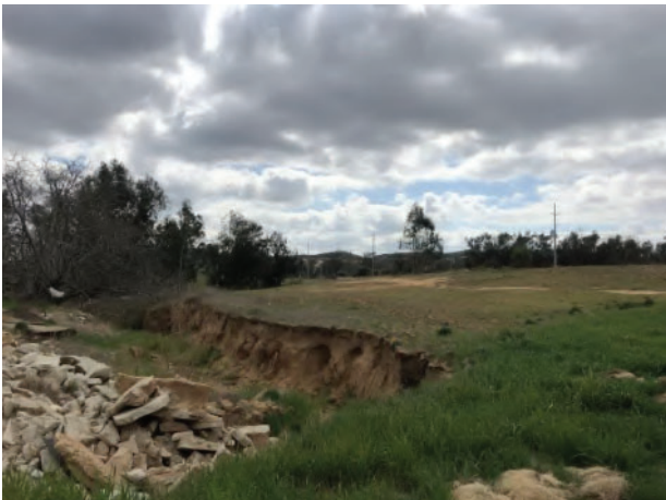
17.View of the south parcel from the east looking southwest.
