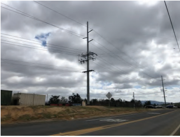
1.View of the subject property from the northwest across Veile Avenue looking southeast.
