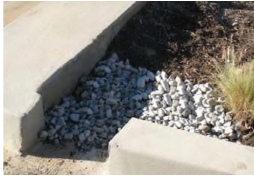
Figure 2: Curb Cut located in a Bioretention Facility
