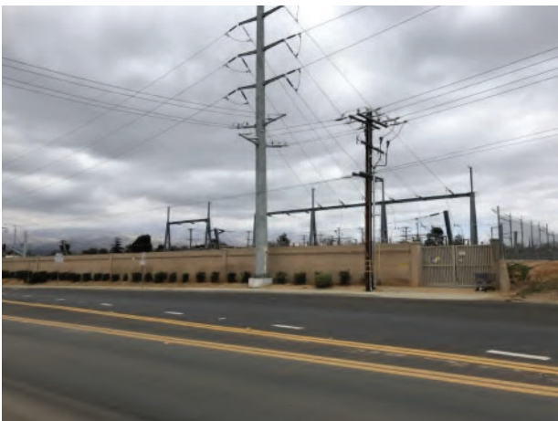
23.View of the adjacent substation to the north.
